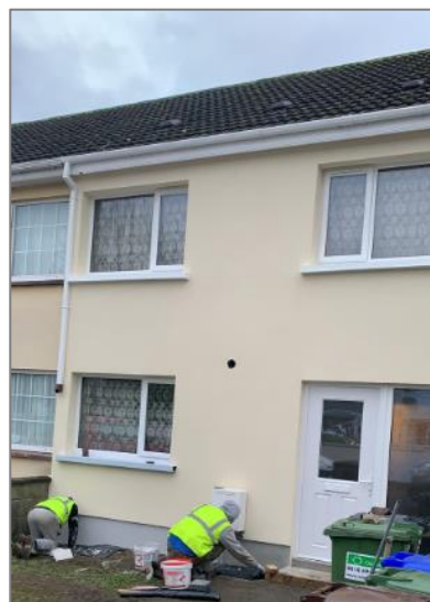
Figure 9: Retrofitting of housing with improved insulation, doors, windows, and heat pumps to improve energy efficiency
