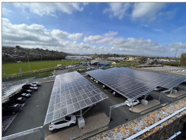
Figure 8: The solar panel covered car park facility in Wicklow that provides 300kW of renewable energy.
